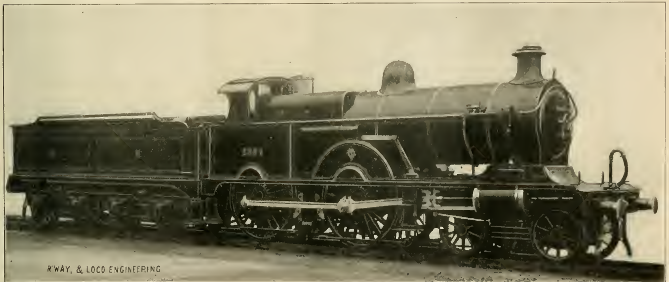
THREE-CYLINDER COMPOUND PASSENGER ENGINE FOR THE MIDLAND RAILWAY OF ENGLAND.
